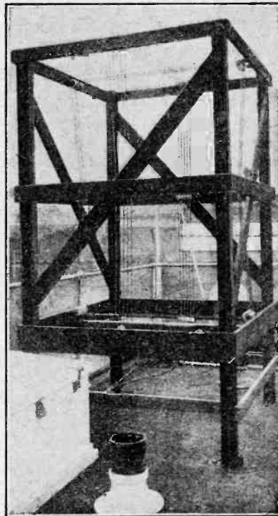
WIRELESS AT THE SHIPPING EXHIBITION. The new Marconi D.F. aerial, now on view at Olympia. Economy of cost and space are both achieved with the new arrangement without sacrificing the accuracy obtainable with a large and unwieldy loop.
